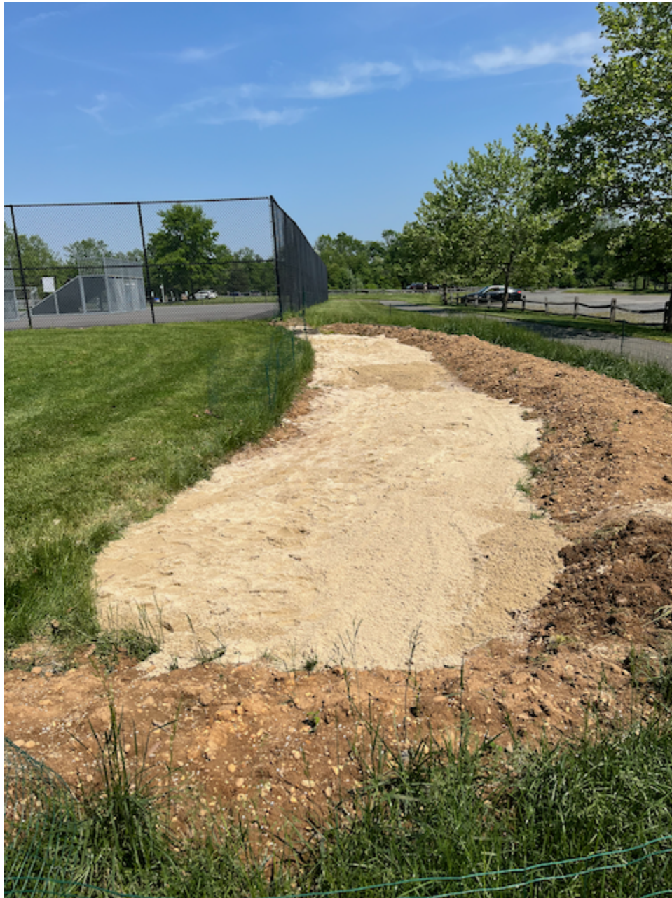
Figure 24: Applying soil amendments
