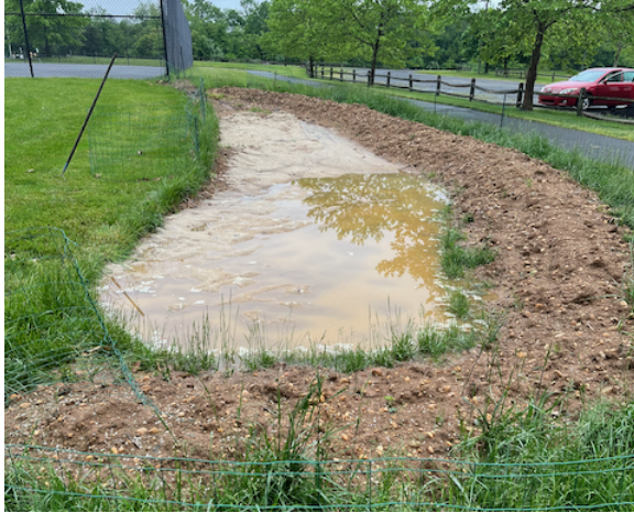
Figure 20: Standing water on the aquifer
