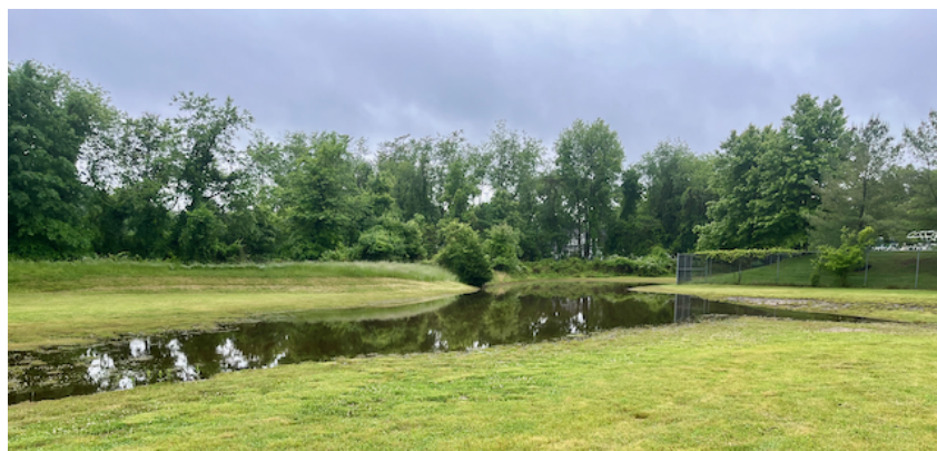
Figure 3: Existing stormwater management basin
