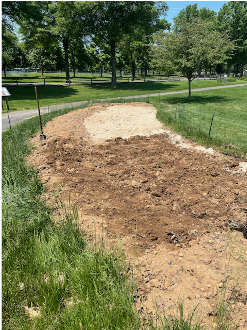
Figure 25: Original soil being added back to garden
