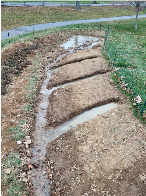
Figure 18: Horizontal sand wicks (left) did not solve the standing water issue (right)
