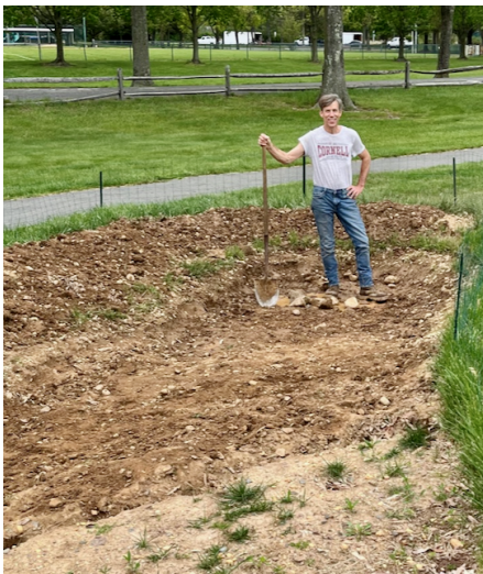
Figure 19: Creating an Aquifer by digging a deep and wide hole (left) and filling it with 13 tons of sand (right)
