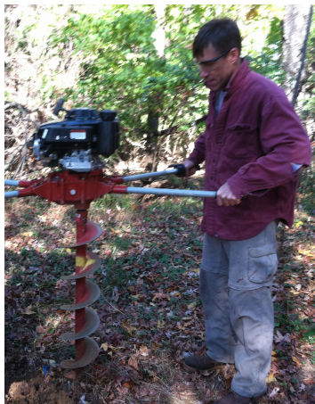
Figure 16: Using an auger to create infiltration “sand wicks”
