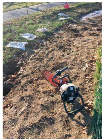
Figure 16: Using an auger to create infiltration “sand wicks”
